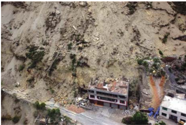
Fig. 6 Landslide buried road and building in Wenchuan County
