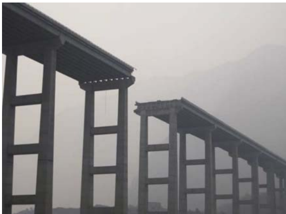
Fig. 14 Damage to the Yingxiu Bridge caused by the falling of one of the central spans. The bridge is located at the upstream of the Minjiang River at Zipingpu Reservoir
