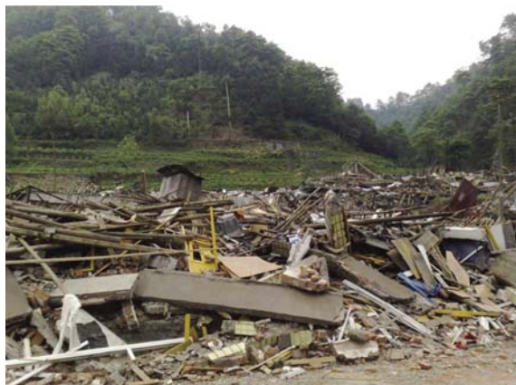
Fig. 6 Complete destruction of Yinghua Town, Shifang City
