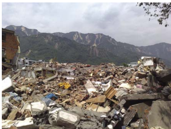
Fig. 5 Complete destruction of four buildings of the Dongqi Middle School in Hanwang Town, Mianzhu City
