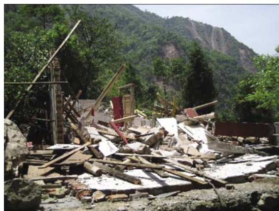
Fig. 7 Collapsed building in a village located halfway up the mountain in Shifang City
