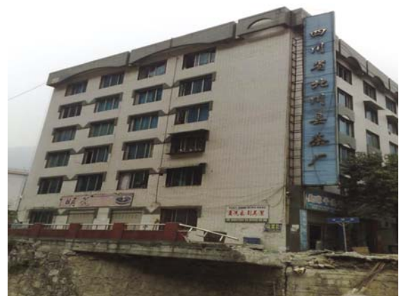
Fig. 22 The office building of Beichuan Tea Factory in Beichuan county town
