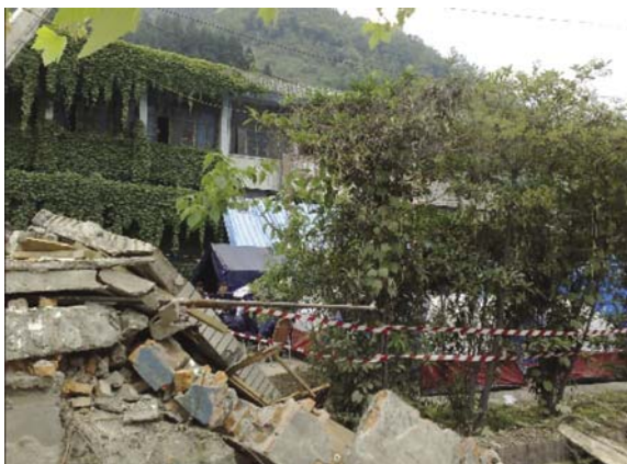
Fig. 25 A one-story building located in mountain region in Shifang City has no obvious damage
