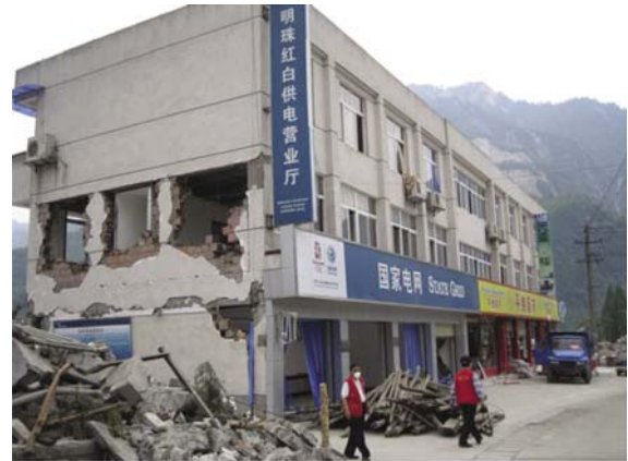
Fig. 21 The only standing building in Hongbai Town, Shifang City
