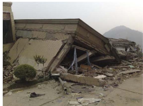
Fig. 12 The upper part of a two-story building destroyed and thrown for a distance of more than 15m
